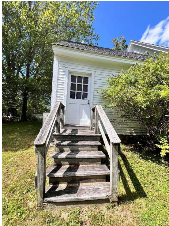
Photo # 4 Side Entrance Door
