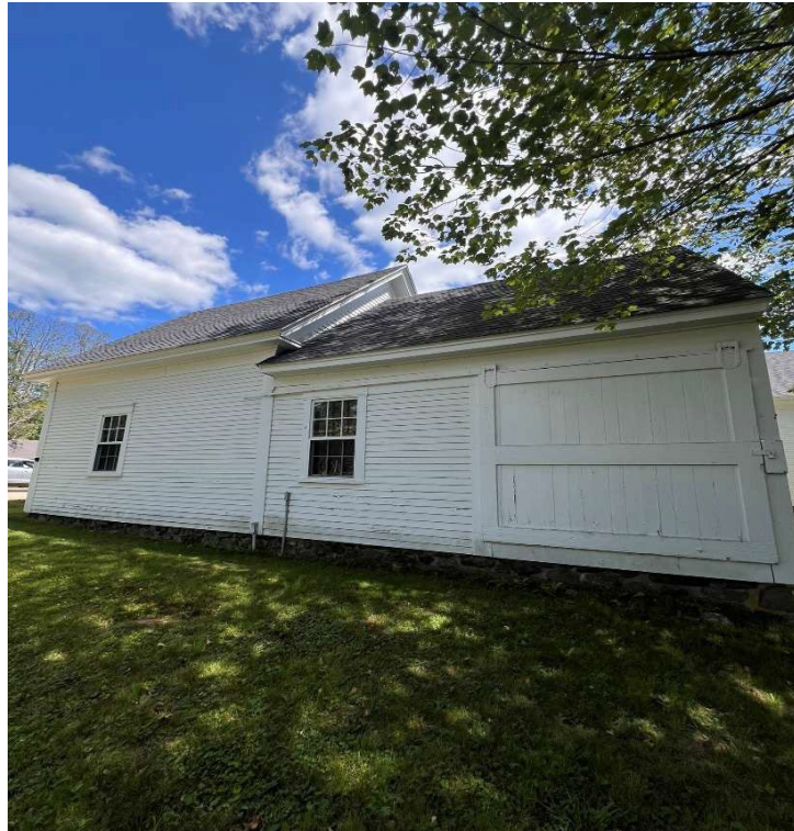
Photo # 2 Right Side looking at the Building, Sliding Door where the Roller would enter/exit on the 1912 addition.
